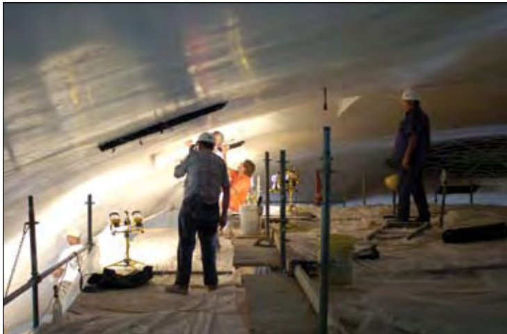
Repairs to the ceiling in Palmer Auditorium were facilitated by a maze of scaffolding that supported a “floor” made for plasterers and other workers.
