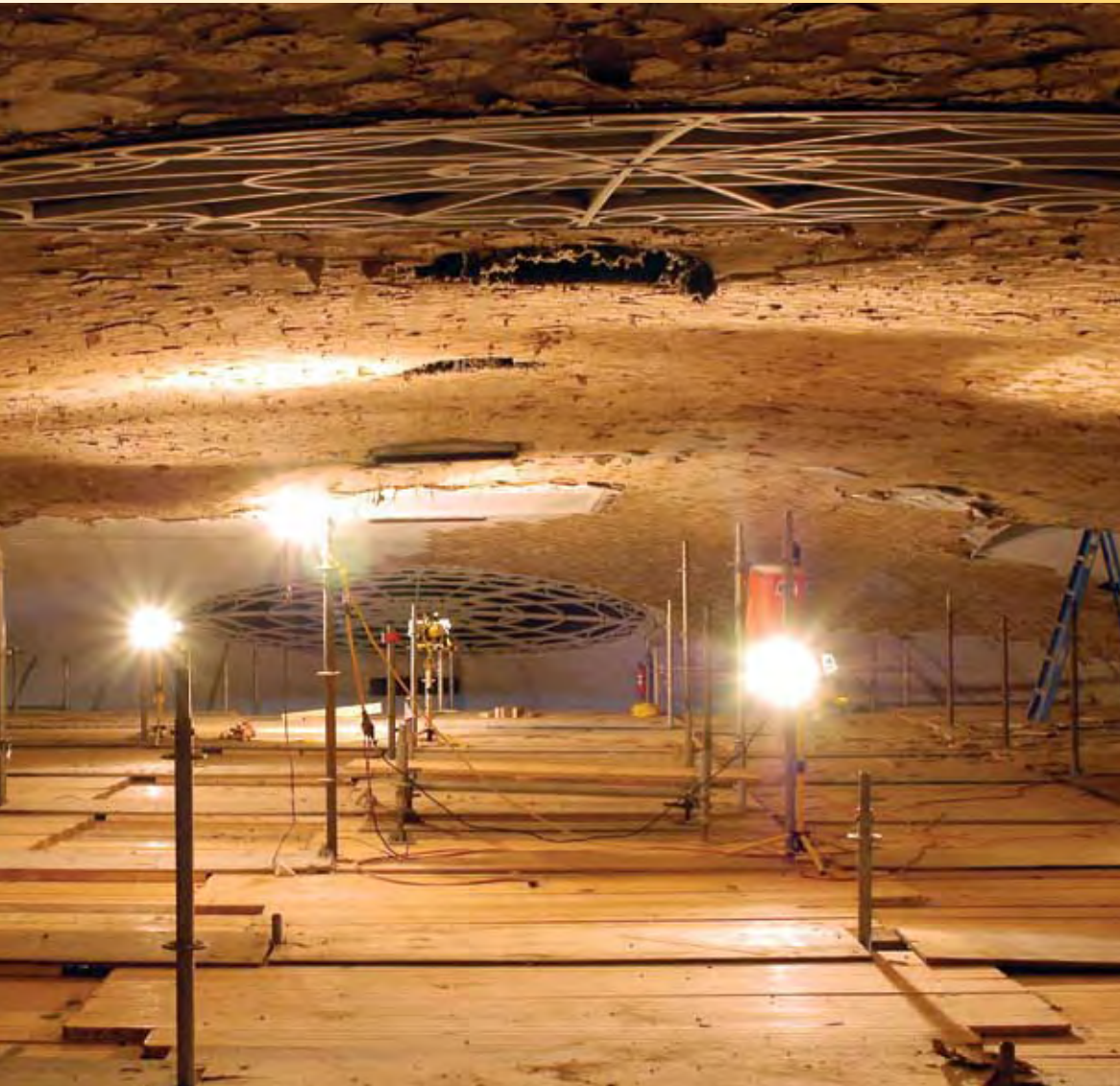
The ceiling of Palmer Auditorium is aglow from work lights that show the extent of repairs that have been in progress this summer. The facility is expected to be ready for occupancy by early November.
